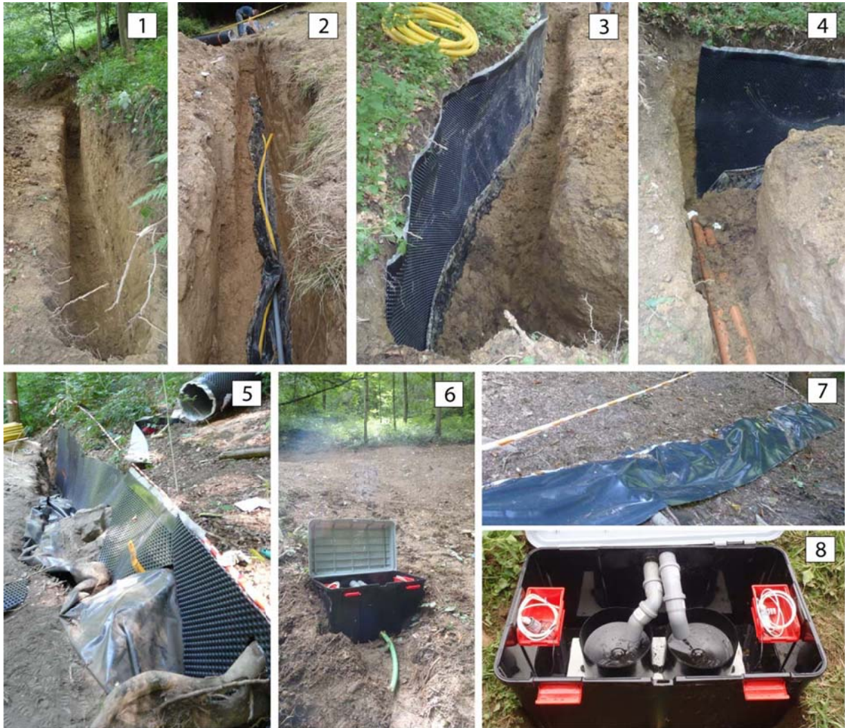
Figure 3: 1) Excavated trench at the forested hillslope; the outlet is on the left side. 2) Trench at the grassland hillslope during the installation of the pond foil, drainage pipe, and solid PVC pipe. 3) Trench after the installation of the drainage mat. 4) Transfer of trench flow into sewer pipes running through the trench outlet. 5) Trench at the mixed forest hillslope after the installation of the drainage system (irregular topography due to bedrock and roots). 6) Location of trench flow measuring box (box with tipping buckets at the end of the sewer pipes). 7) Surface pond foil routing surface flow over the fissure where the drainage mat meets the soil surface. 8) Trench flow measuring box: water from the left and right part of the trench is channeled into tipping buckets with attached HOBO event loggers, and out of the box.
